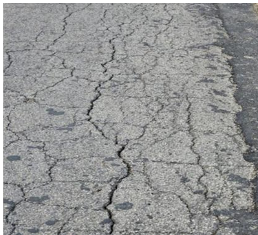
Figure 11: Existing asphalt (axis 3) Figure 12: Cracks and deformations of the asphalt
