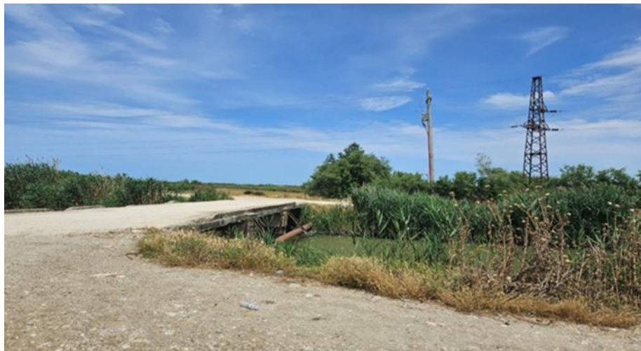
Figure 9: The old bridge (km 3+660)
