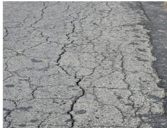
Figure 11: Existing asphalt (axis 3) Figure 12: Cracks and deformations of the asphalt
