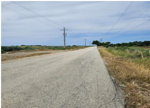
Figure 11: Existing asphalt (axis 3) Figure 12: Cracks and deformations of the asphalt
