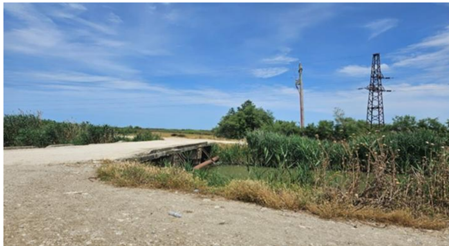
Figure 9: The old bridge (km 3+660)
