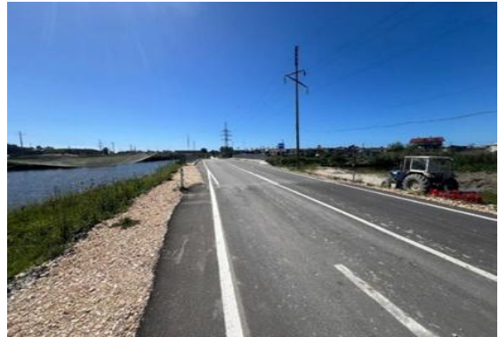
Figure 14: Seg.no.4 recently asphalted with a width of 6m+ stabilizer bank
