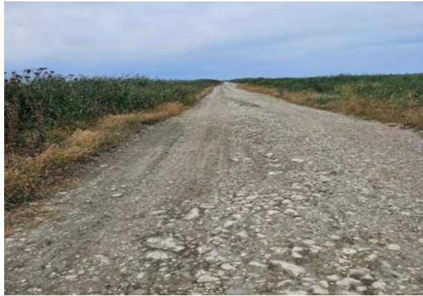
Figure 5: Mixed road materials (axis 1)
