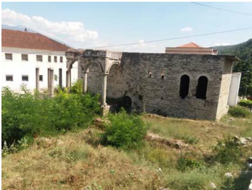
Existing condition of surrounding are of former Selamllik Vrioni
