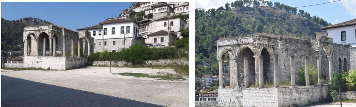
Existing condition of the former Selamlik of Vrioni
