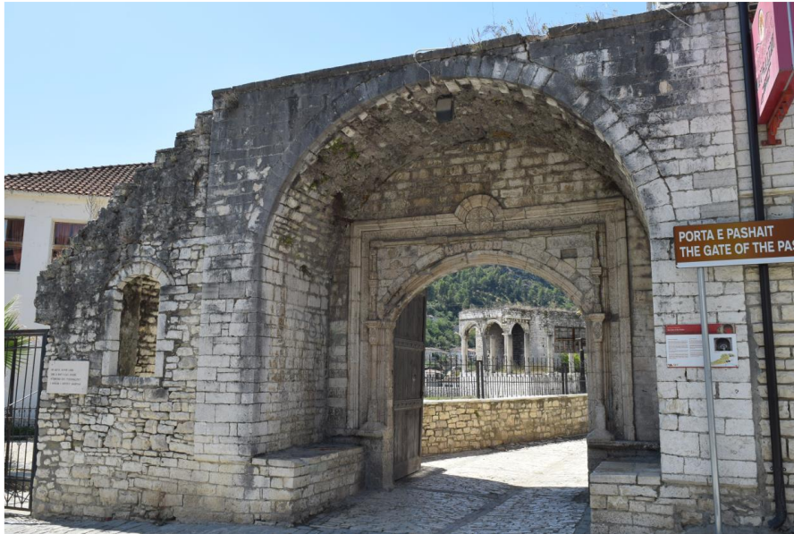
Existing condition of The Gate of Pashai
