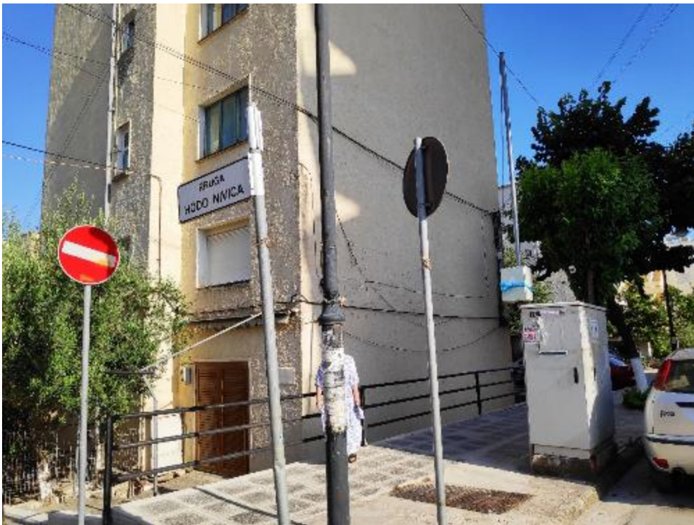
Figure 16 Lack of Safety in Pedestrian Spaces
