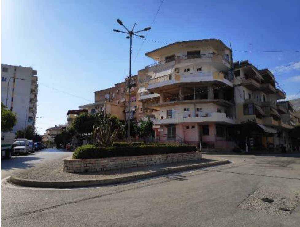
Figure 15 Photo of the Existing Layout of the Square
