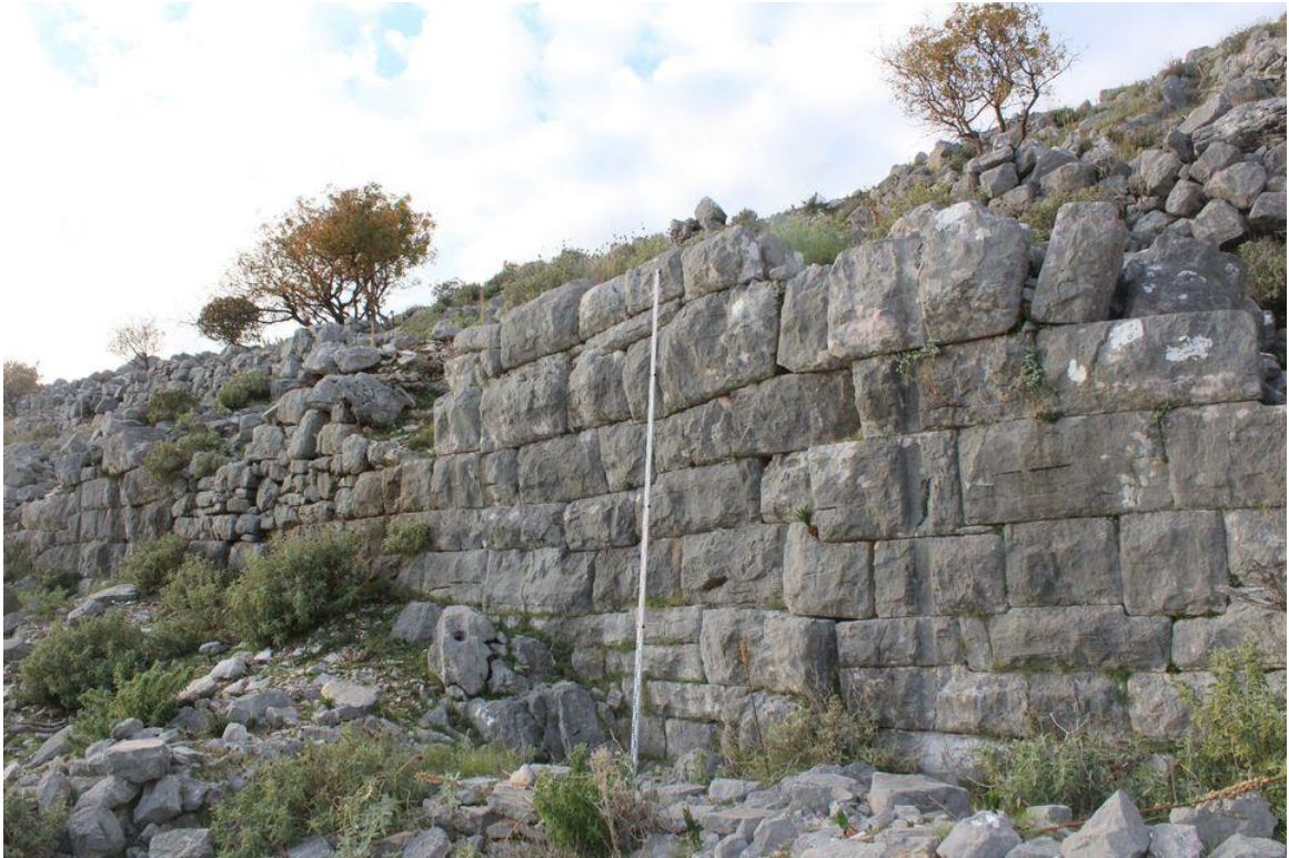
Figure 10 Walls with stone blocks of the ancient period (NICH Vlora)
