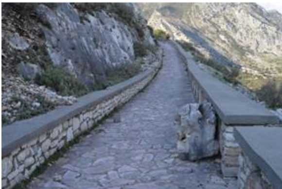
Figure 27 Detachment of the rock material from the slope (NICH)
