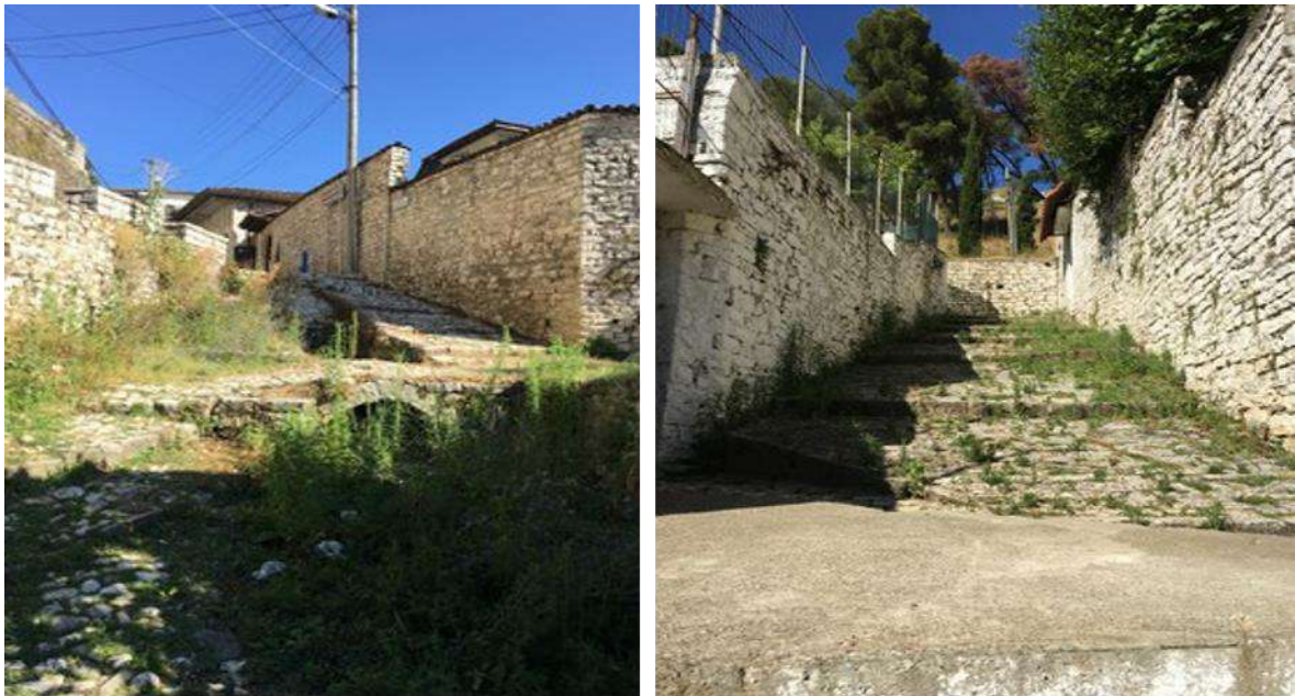
Figure 23. Toli Bojaxhiu street, decay of the horizontal surfaces
