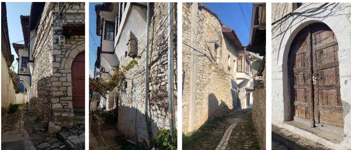
Figure 33. Individual residential building on “Llambi Guxhumani” street
