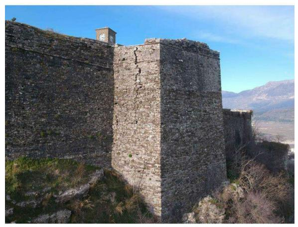
Figure 36. Cracks in walls
