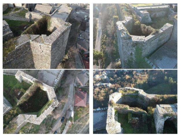
Figure 39. Aerial views of the model. Interior thinner walls are the original defensive walls and the thicker exterior walls
