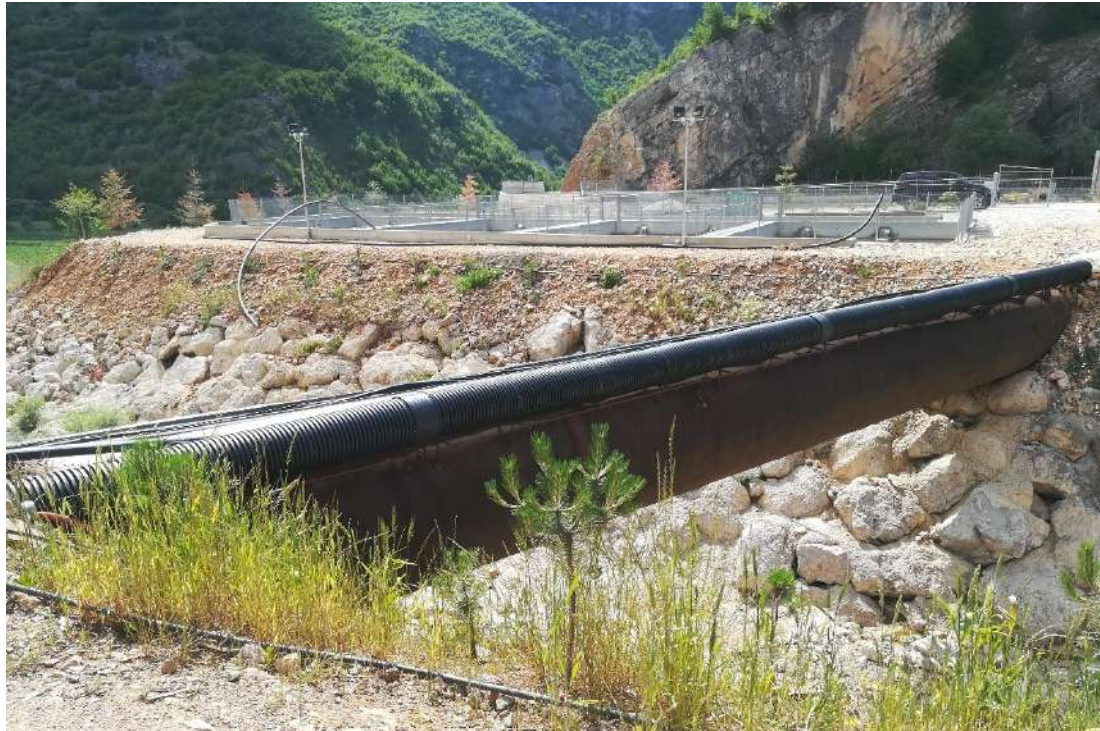
Figure 3-7: Privately owned Hydropower plant (near Borove and within the working width)
