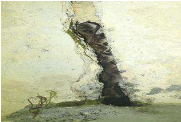
Figure 4-25 Unidentified species under bridges at Sites 9 and 10
