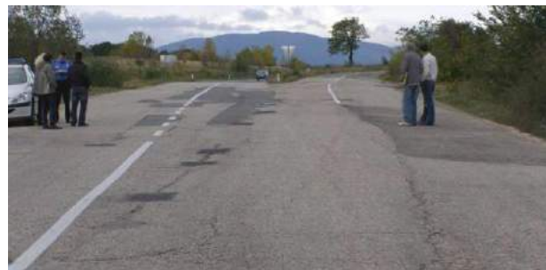
Dangerous "Y" type intersection
