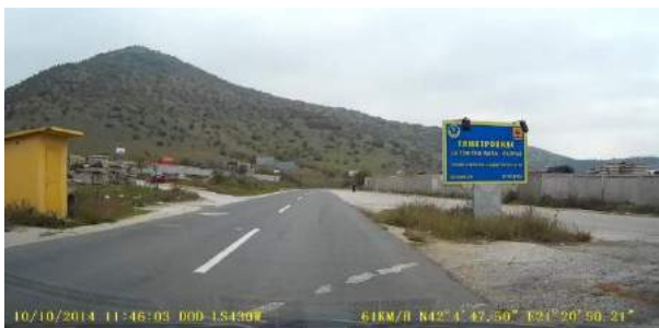
Missing access control (Route 6)
