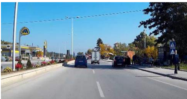
Pedestrian crossing over four lane carriageway
