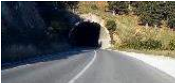
No lights in tunnel
