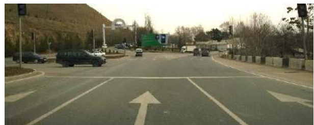
Missing channelisation in junction
