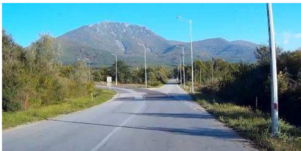
Dangerous "Y" type intersection
