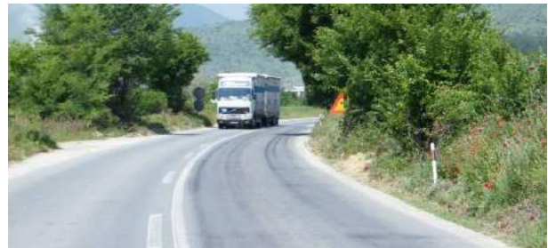
Insufficient site distance in curve
