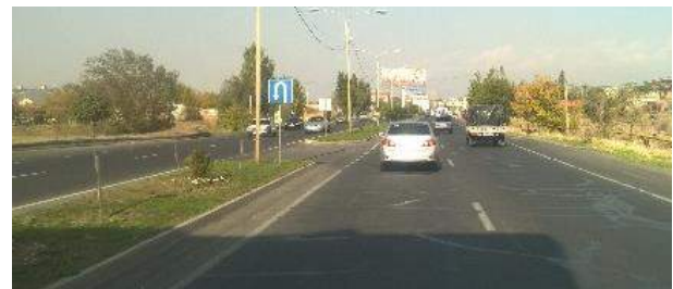
Danger place for U-turn
