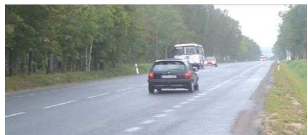
1+1 road with wide (asphalted) hard shoulders
