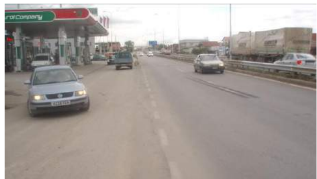
Services along road
