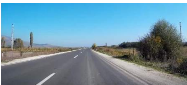
Too wide traffic lanes
